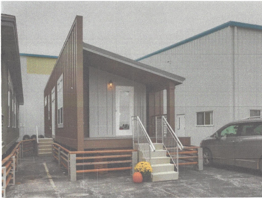
Look Out Lodge SG55 Exterior Photos
